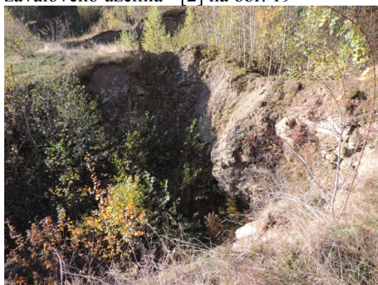
Obr. 24: Detail závalu - bod [3] na obr. 19
